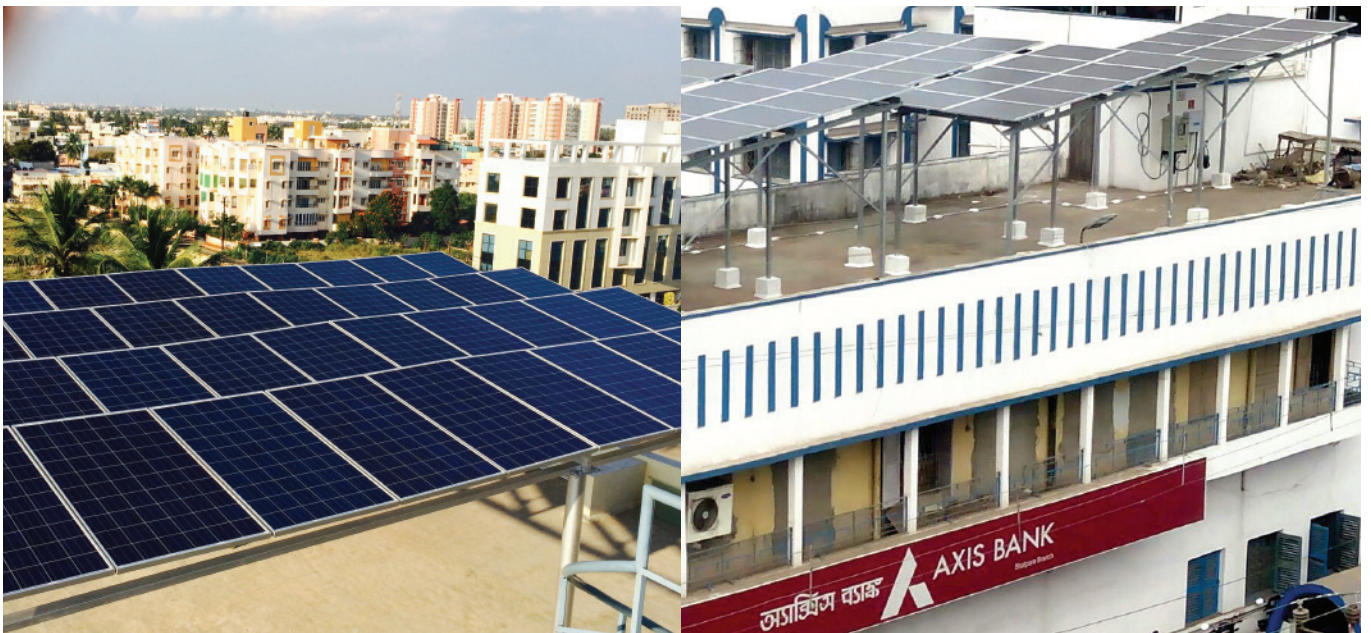
Solar panels installed at the Bank's branches
